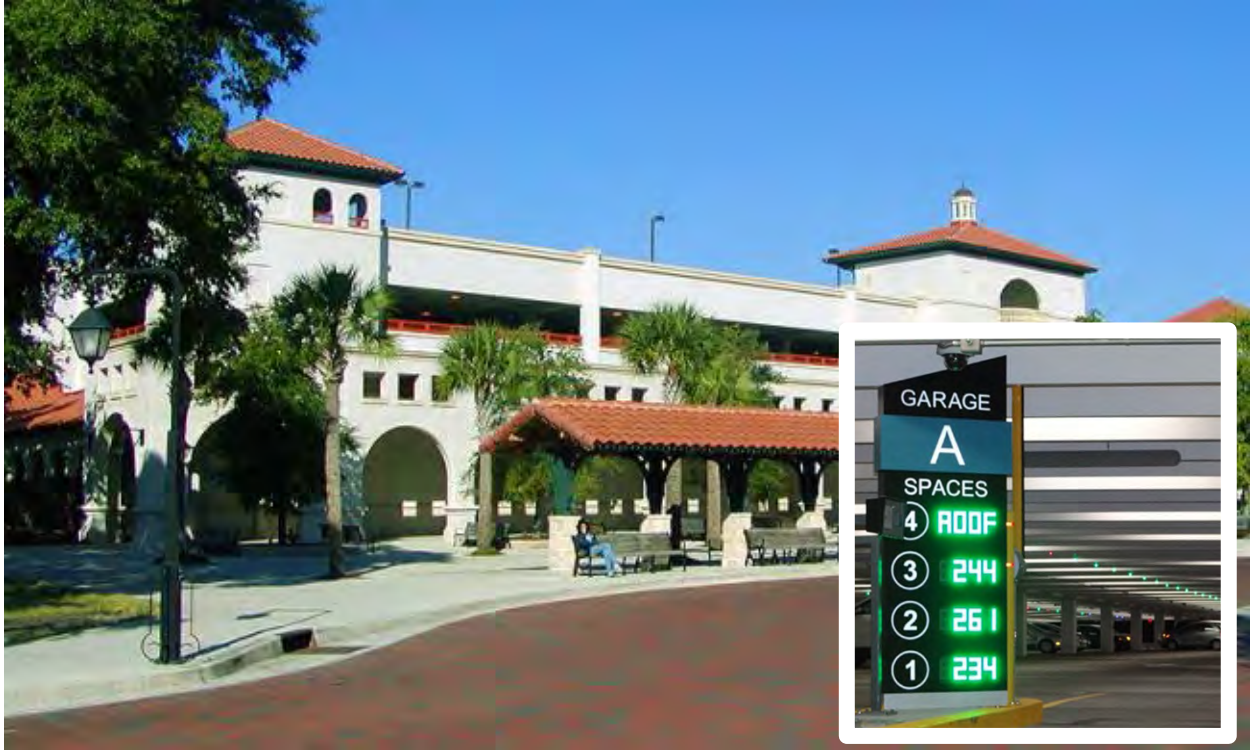
Figure 43. Historic Downtown Parking Garage
